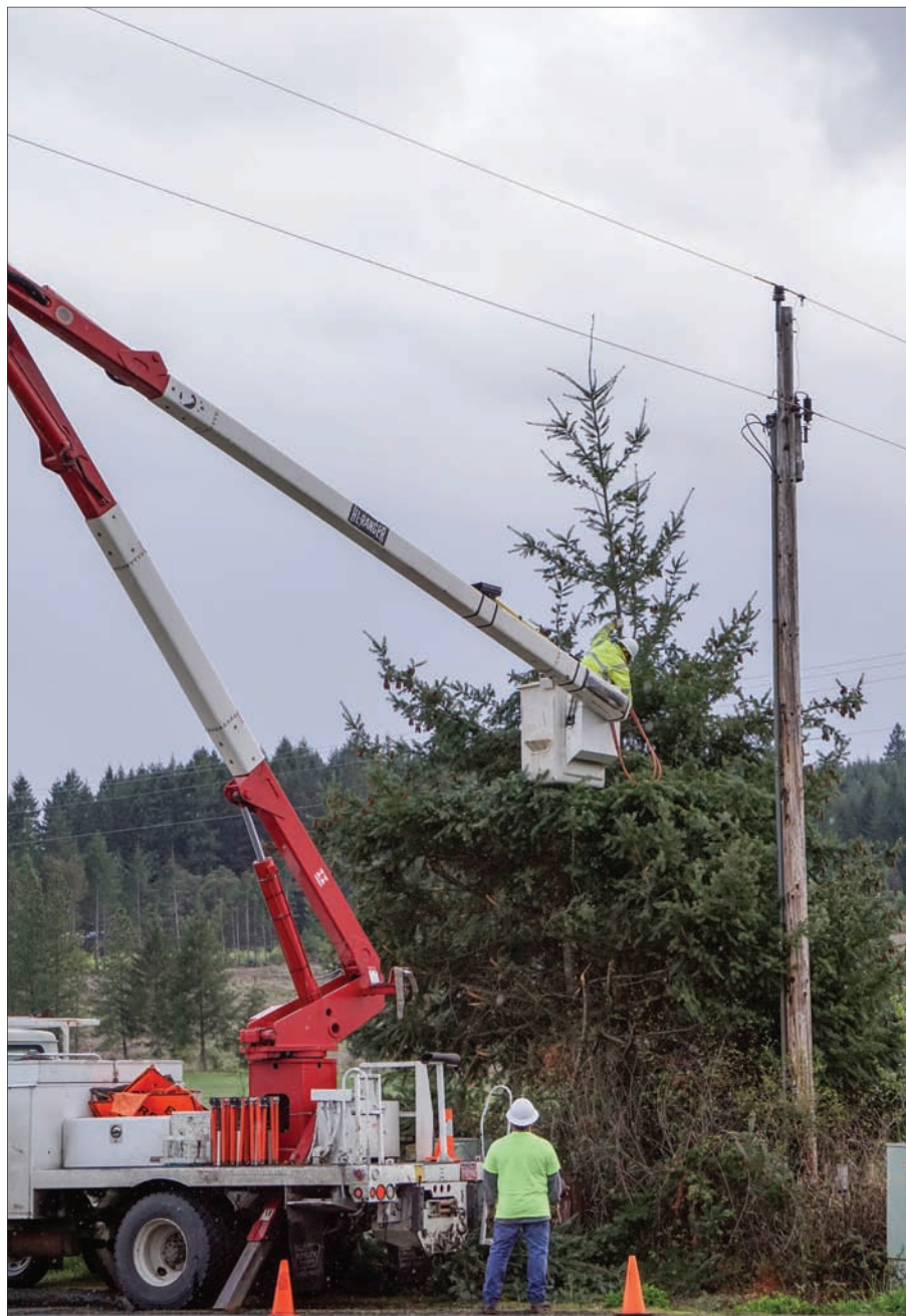
Trees growing too close to power lines can cause outages, so a Blachly-Lane crew trims or removes trees that are potential hazards.
